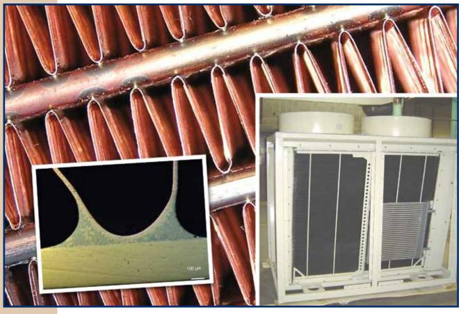
Young Touchstone used the *Cu*proBraze process to braze these serpentine copper fins to flat brass tubes for this locomotive charge air cooler application. The electrochemical potential is about the same for the fins, tubes and filler material so there is little tendency toward galvanic corrosion.
